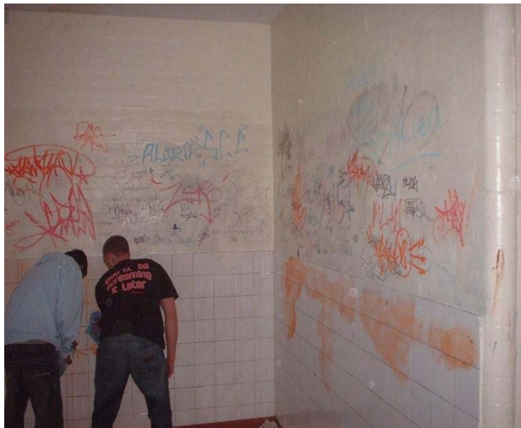
Painting out graffiti in the toilet block, Frome college
